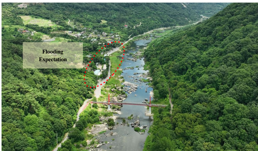
Fig. 5. The access road to JangGun-Mok (Operational constraint)
